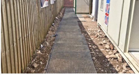
Housebuilding: Clean, safe walkways on-site.
