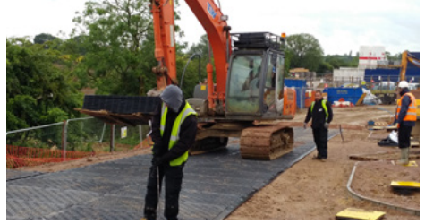
Construction: Supporting heavy vehicles and cranes.
