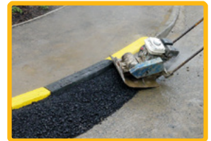
Haunch with temporary tarmac
